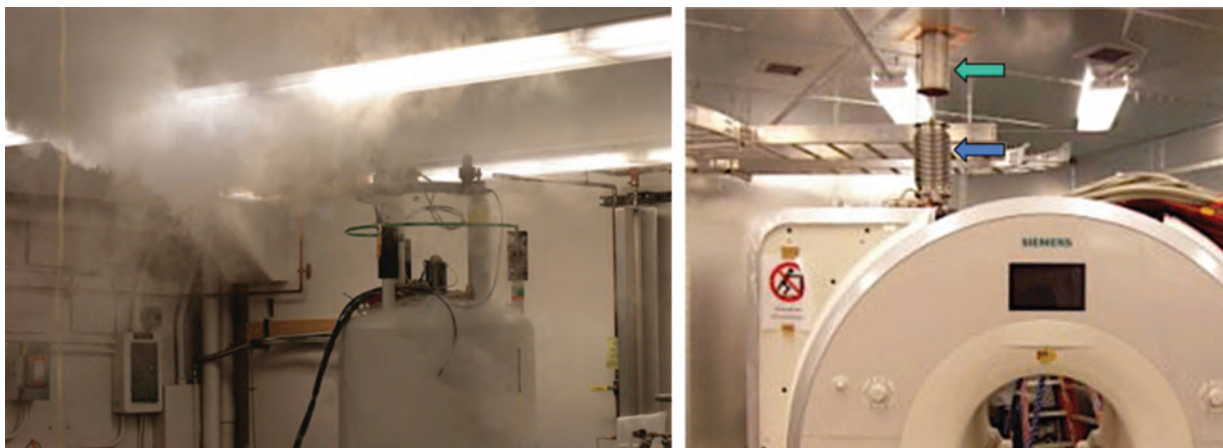
Figure 2. A quench event in a research MRI magnet (left) shows the release of gaseous helium. Such events necessitate stringent safety protocols, including appropriate ventilation systems and emergency procedures to protect personnel from cryogenic hazards and asphyxiation risks. In an installation of a quench tube in an MRI (right), the blue arrow points to the tube and the green arrow points to the vent in the ceiling. Quench tubes serve a crucial role in venting helium gas from the MRI scanner during a quench event. Proper attachment and secure connections between the quench tube and vent are vital to maintaining safety within the MRI suite, especially during quench scenarios. Printed with permission from MRIquestions.com.
