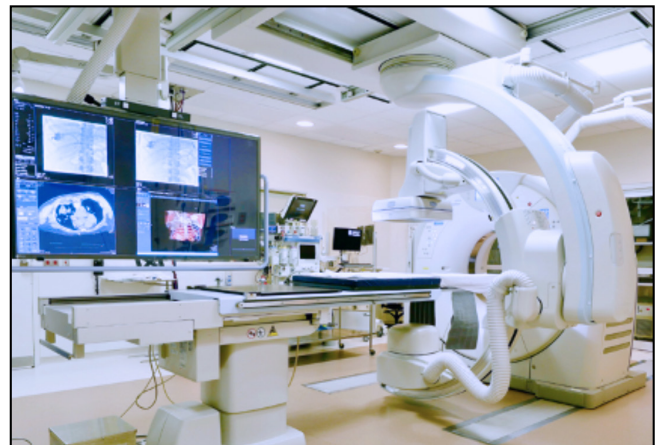
FIGURE 1. The hybrid angio-CT (Canon 4D CT) system combines a CT scanner and an interventional angiographic c-arm in the same lab.
