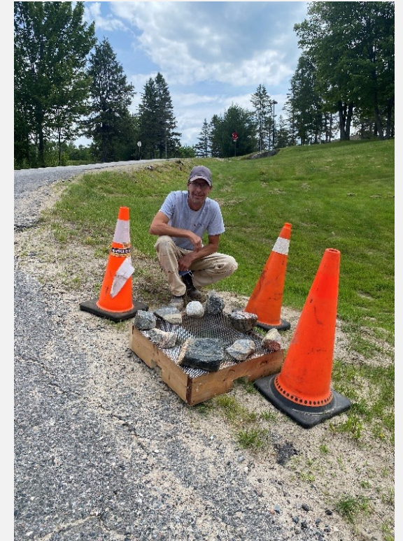
Maintenance & Facilities Department at College Drive Campus
