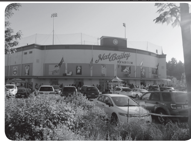
An outside view of Nat Bailey Stadium.
