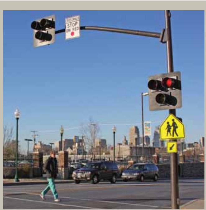
KCUMB recently installed a new pedestrian crosswalk along Independence Avenue, making it safer for students to cross the busy, four-lane street. The crosswalk flashes red when activated by a pedestrian.
