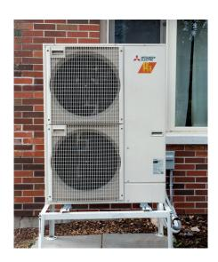
The Zuba Central system is the perfect solution for our cold Canadian climate. Performing best at low temperatures, it provides 80% of its rated heat at -25°C, meaning it operates superior to other central heat pumps. Thanks to this much heat being generated efficiently at low temperatures, the inefficient backup electric heaters will rarely be used, if at all. The Zuba Central also provides efficient cooling.
