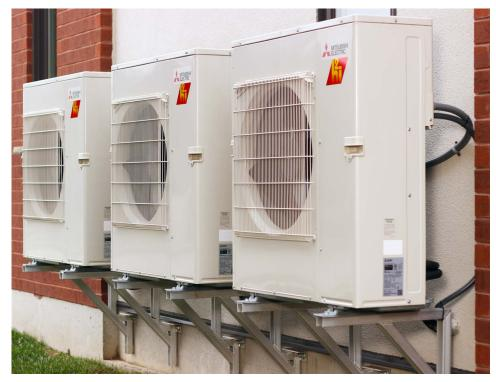
Part of the Zuba family of Mitsubishi Electric products, the centrally ducted cold climate air source heat pump system chosen features 100% output at -15°C, which is substantially better than previous product in phase 1.
