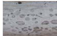
No Dual Barrier Coating Used
